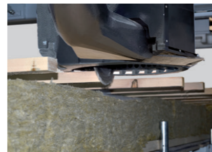
Formatting the roof battens
